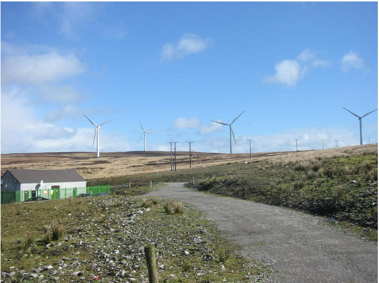
Figure 1 - General view of Tappaghan wind farm control room/sub station and the four closest turbines.
