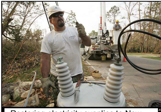
Restoring electricity supplies to New Orleans after Hurricane Katrina. (picture courtesy of USA Today.)
