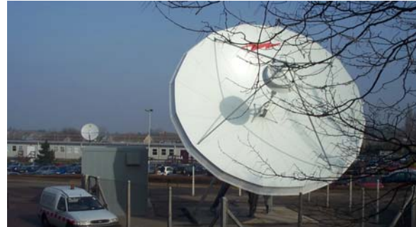
7.5 metre satellite dish serving as a hub for a private VSAT network in a UK utility.
